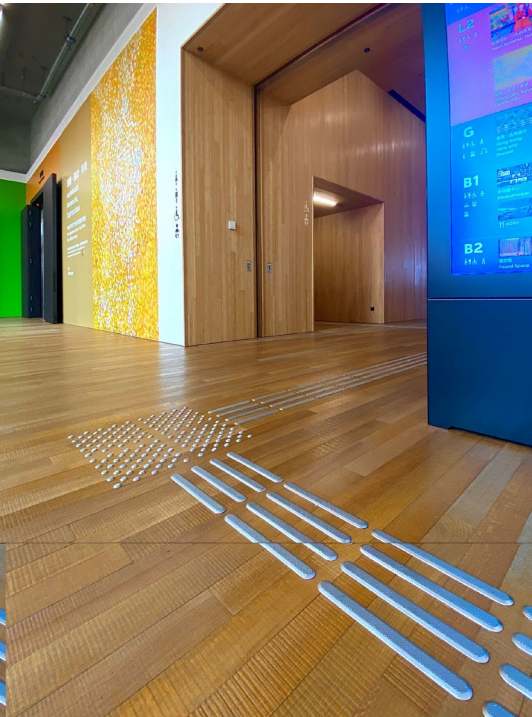
Tactile guide paths leading to the accessible toilet
