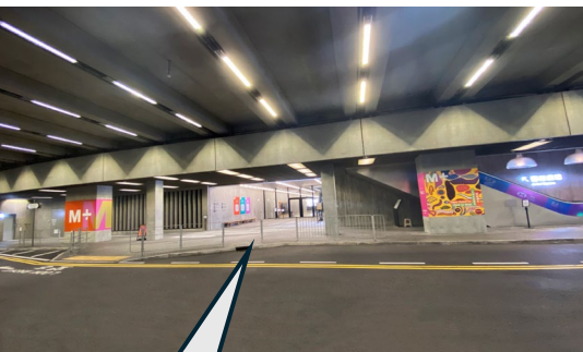
B1/F Cultural Drive Entrance
