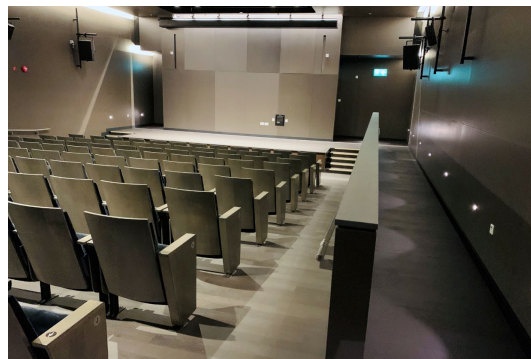
FHKA Seminar Hall ( 2/F ) was designed with a stepless route for accessing from the auditorium to the stage
