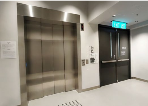
G/F lift lobby
